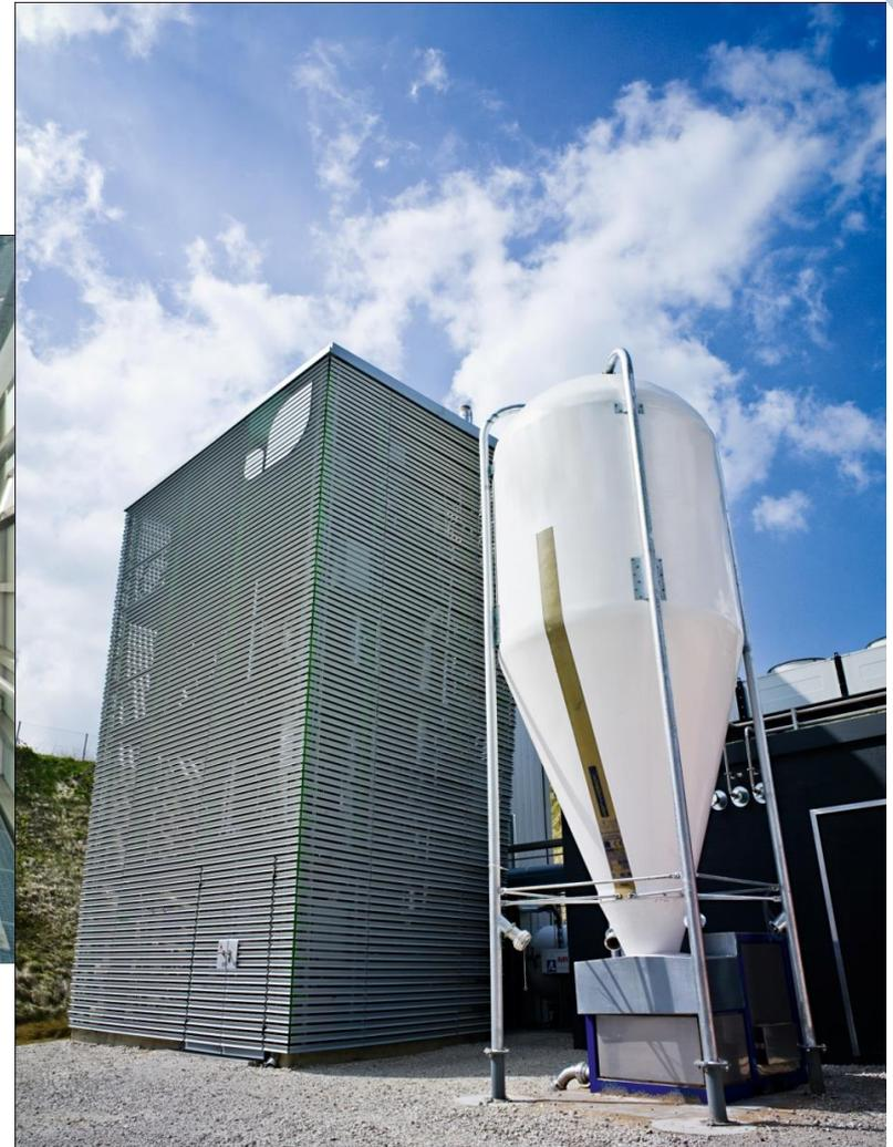
Agnion Heatpipe Reformer Technology for small scale application (e.g. 0,5 - 1 MW<sub>el</sub>)
